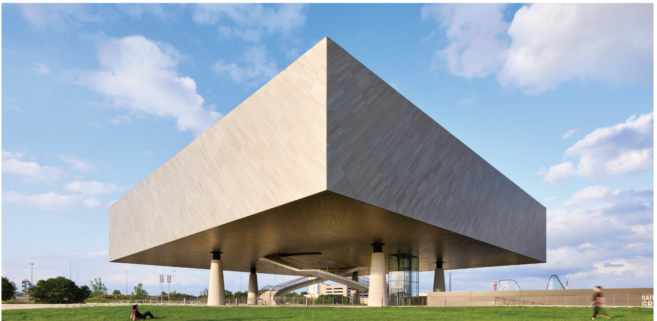
The project team for the National Medal of Honor Museum in Arlington, Tex., initially considered supporting the monolithic building with full-height precast concrete columns. Through engineering analysis, the precast concrete specialty engineer determined that only hollow columns could meet all load requirements while accommodating utilities. © Corey Gaffer Photography.
