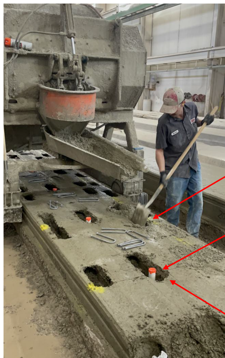
Figure 7. Step 4 in the embedded plate and stud installation process, where the void and removed flanges are backfilled after inserting the hardware. The flat portion of the embedded plate is sitting on the formwork bed, and the top of the polyvinyl chloride (PVC) pipe remains exposed on the top side of the slab.
