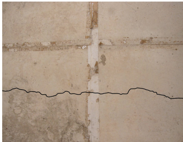
Transverse cracks typically observed on the soffit of the reinforced concrete deck slab between girders
