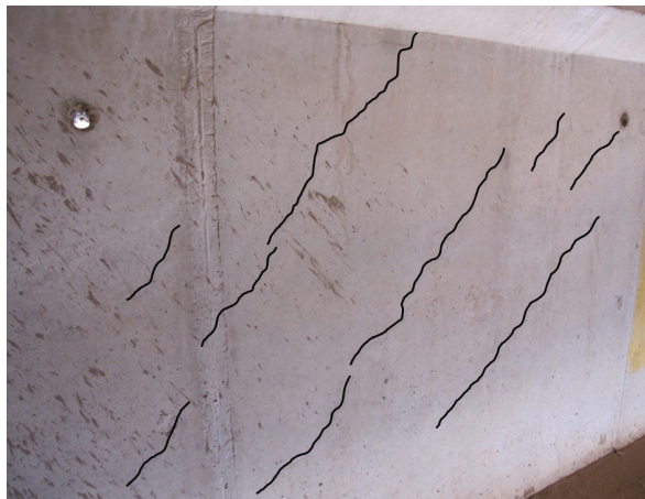
Inclined cracks in the web of a prestressed concrete girder near its ends
