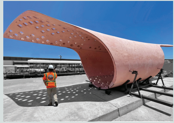
Figure 2. Architectural students designed this complex, ultra-high-performance concrete prototype shelter using precast concrete components. Source: Reproduced from PCI Design Handbook: Precast and Prestressed Concrete , ninth edition (Fig. 1.2.57).
