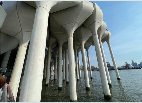
Figure 1. Precast concrete piles and flower pots solved construction and durability issues for both the contractor and owner of this coastal park structure. Source: Reproduced from PCI Design Handbook: Precast and Prestressed Concrete , ninth edition (Fig. 1.2.56).
