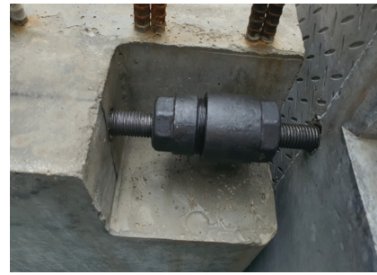
Beam-column splice
