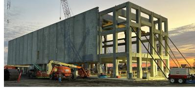
Tindall Corp.'s advancing bar connector system of custom-engineered structural members spliced together with NMB Splice Sleeves' reinforcing bar coupler greatly accelerated project delivery for new insulated substation buildings on the Gulf Coast by using emulative design concepts. Courtesy of Cajun Industries LLC.
