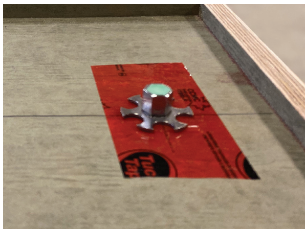
Headed insert affixed with double-sided tape
