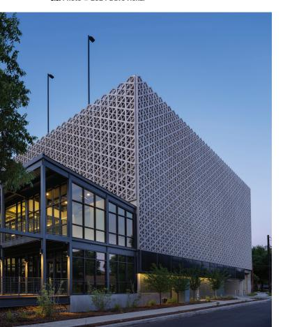
GVI to accomplish this via custom-designed architectural precast concrete panels with a pattern of triangular openings.
