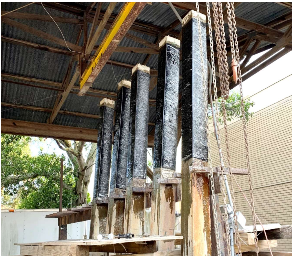
Figure 18. Repaired piles with stretch wrap removed (24 hours after repair).
