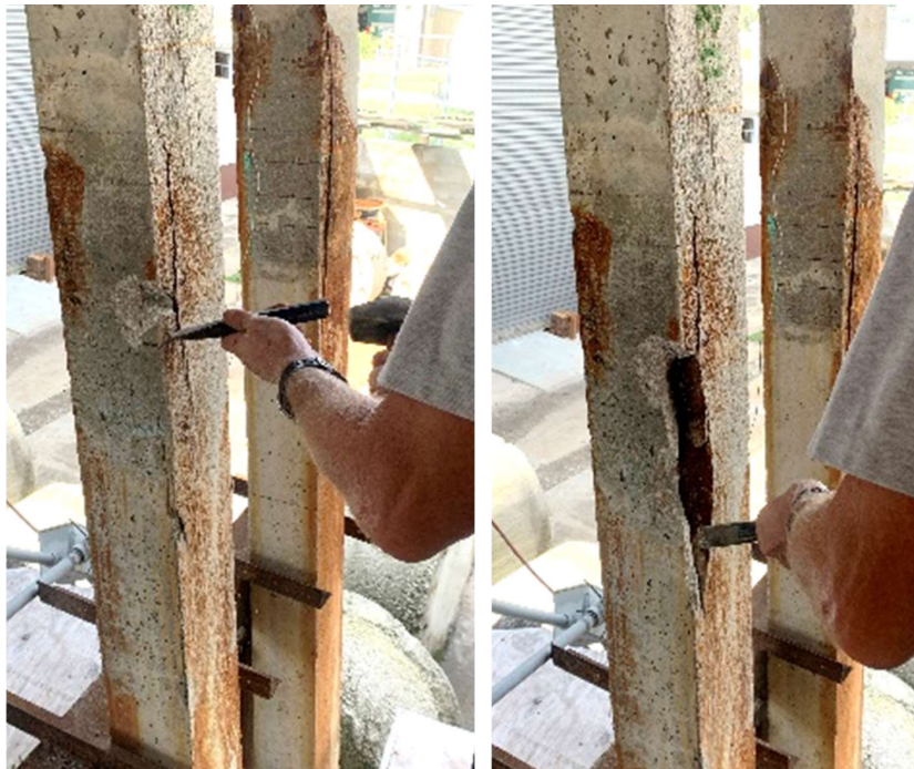
Figure 8. Concrete cover removal of pile 3, which was originally intended to be repaired by epoxy injection.
