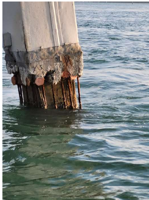
Figure 2. Structural pile jacket repair installed circa 2021 and the same pile, three years later.
