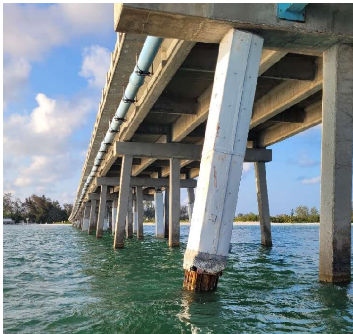
Figure 2. Structural pile jacket repair installed circa 2021 and the same pile, three years later.
