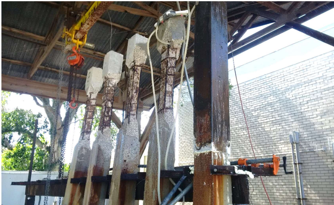
Figure 11. Restored cross section kept wet with soaker assembly dripping down all faces.
