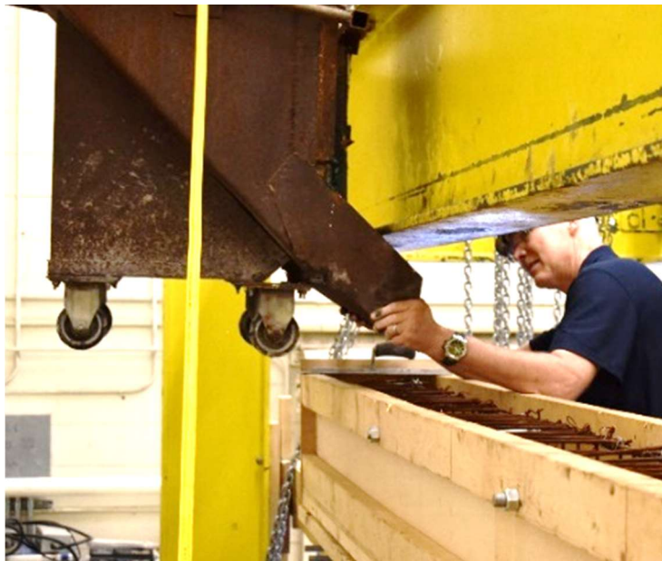
Figure 20. Side discharge concrete bucket suspended above the pile cap.
