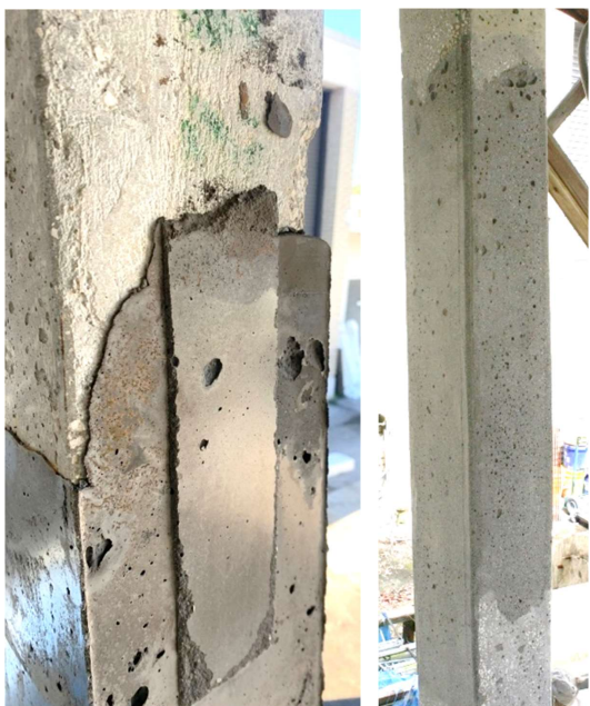
Figure 13. Restored section before and after surface finishing.
