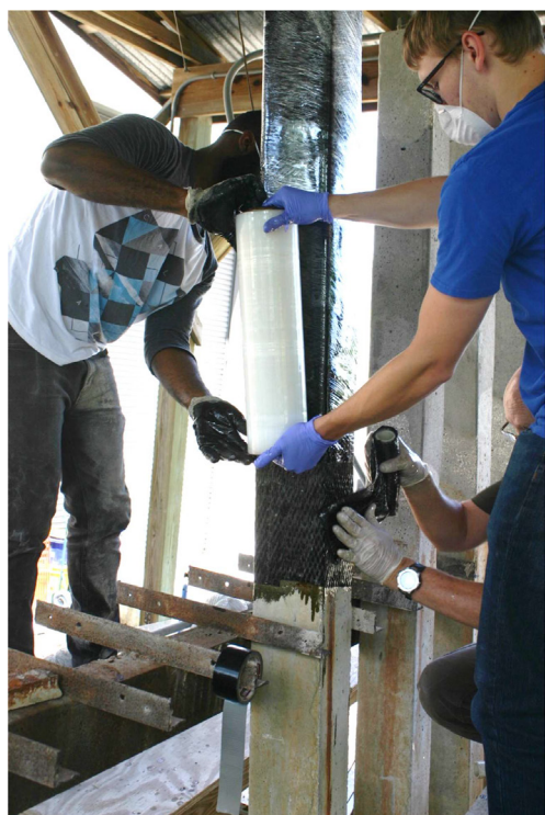
Figure 16. Application of stretch wrap.
