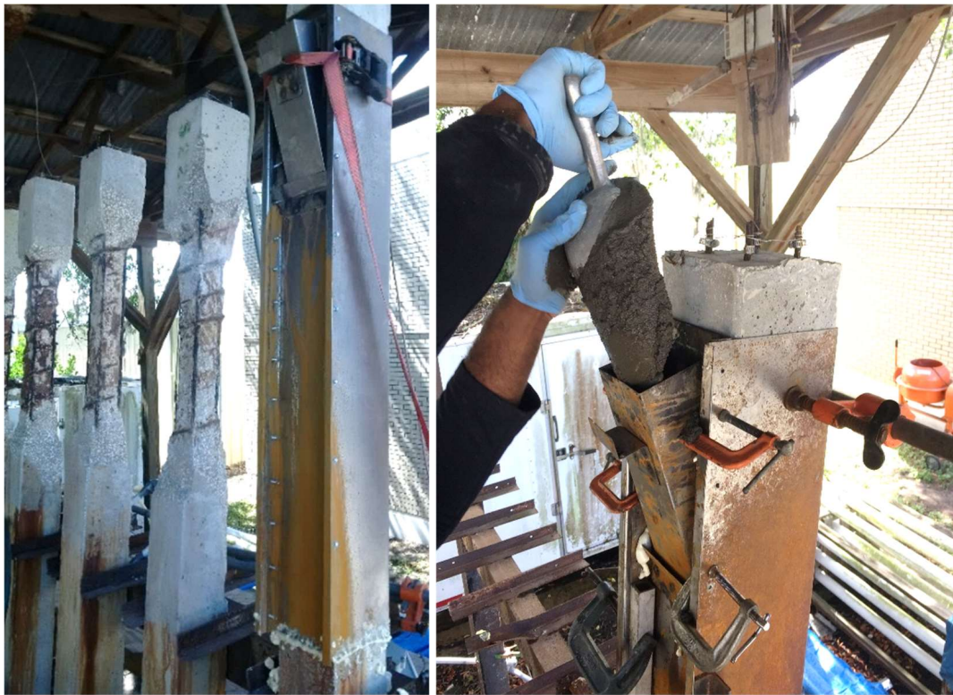
Figure 10. Sheet metal form secured to a pile and filling the form.
