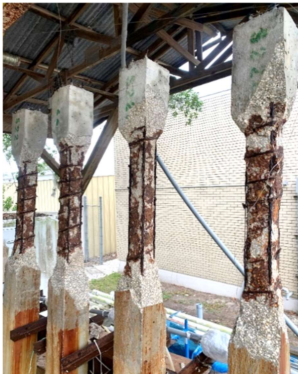
Figure 9. Condition of piles immediately after cover removal.
