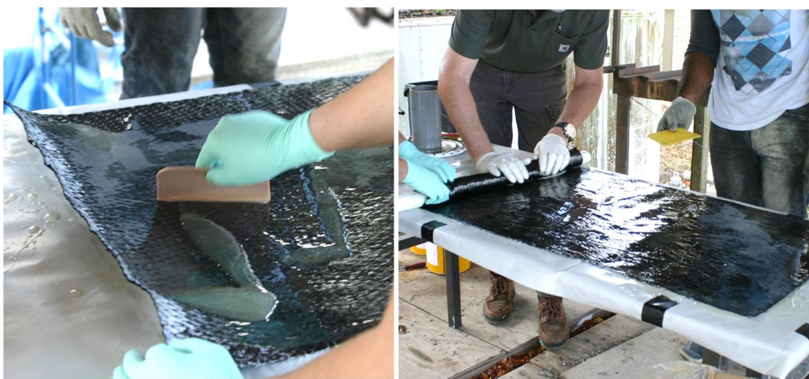
Figure 14. Saturating and rolling the 1.2 × 0.63 m (48 × 25 in.) longitudinal fabric (fibers run from left to right).
