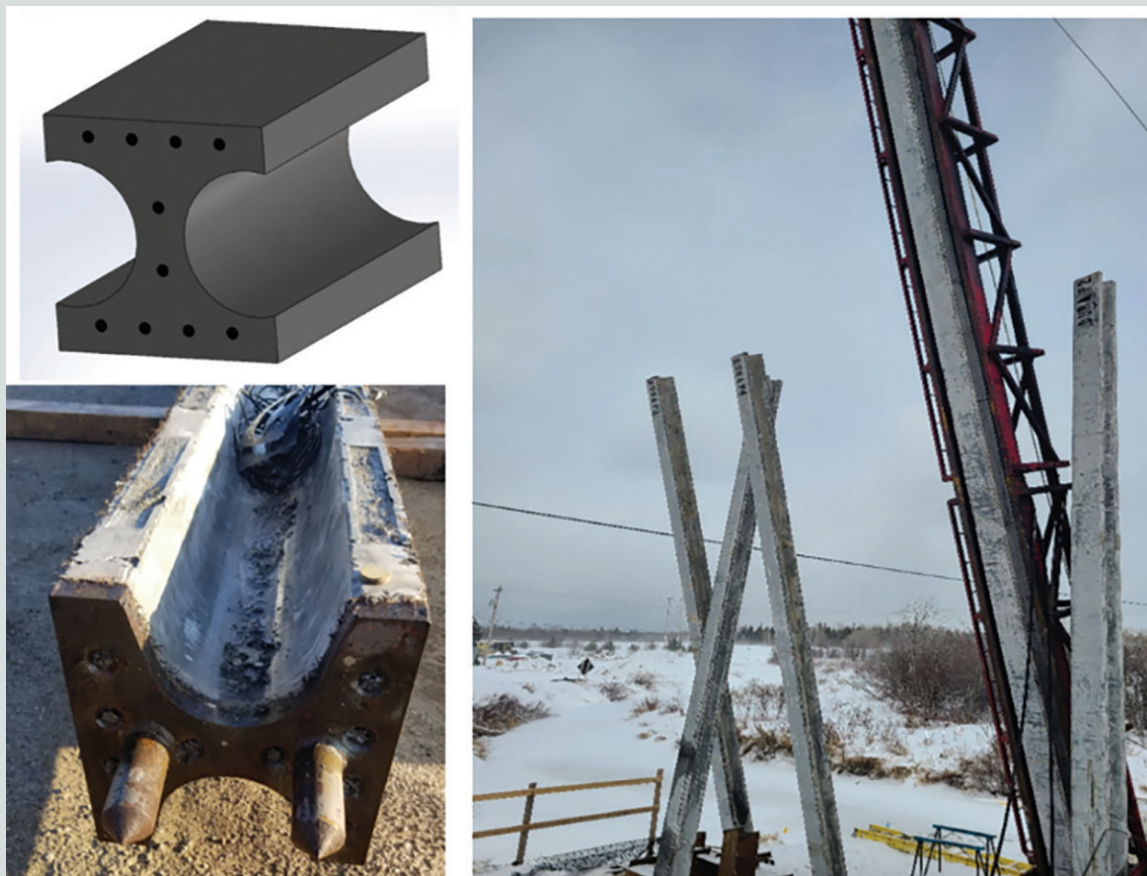
Figure 6.1. Ultra-high-performance concrete battered pile with steel shoe driven by Facca Inc. in Ontario, Canada.
