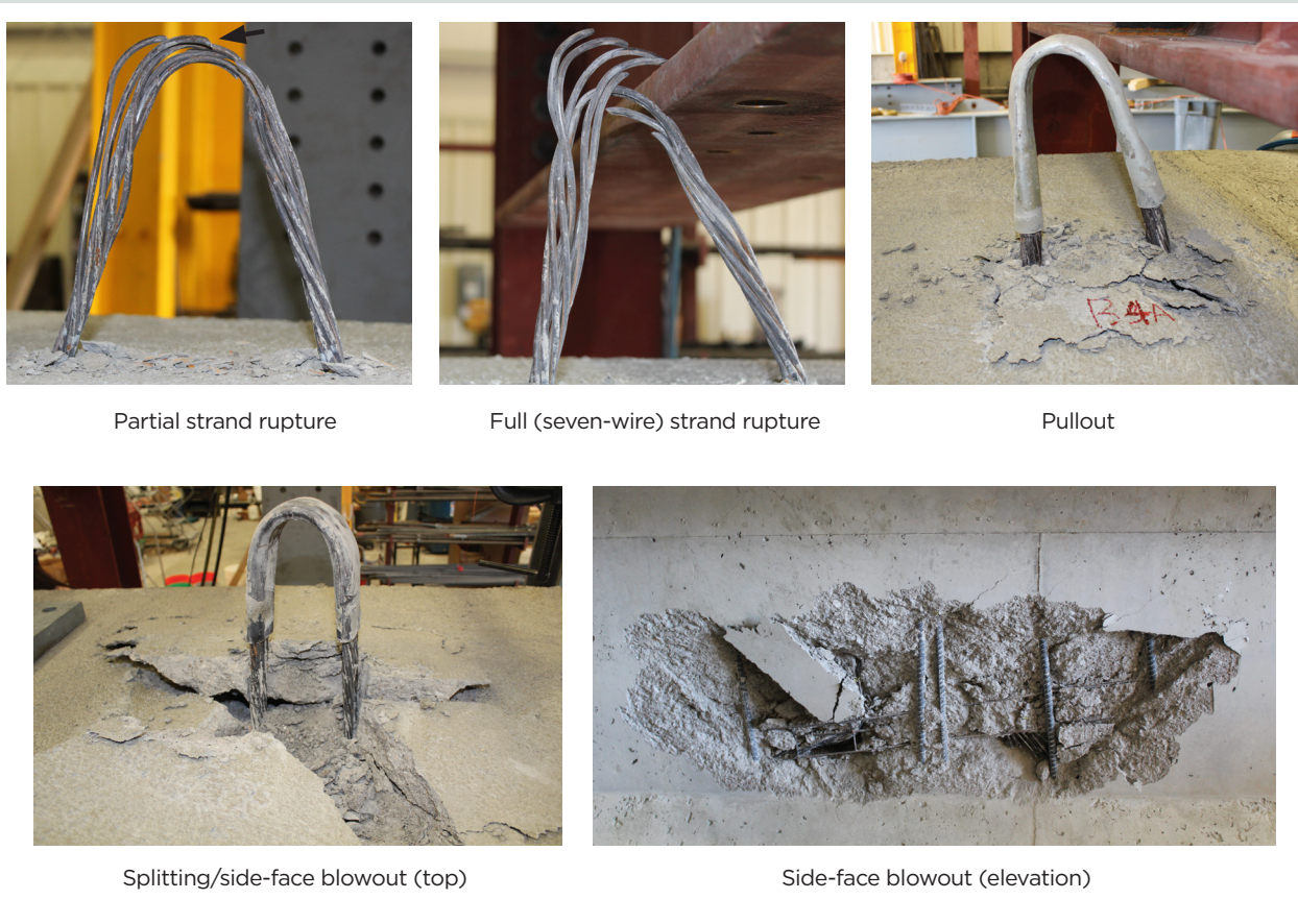
Figure 8. Typical failure modes observed.
