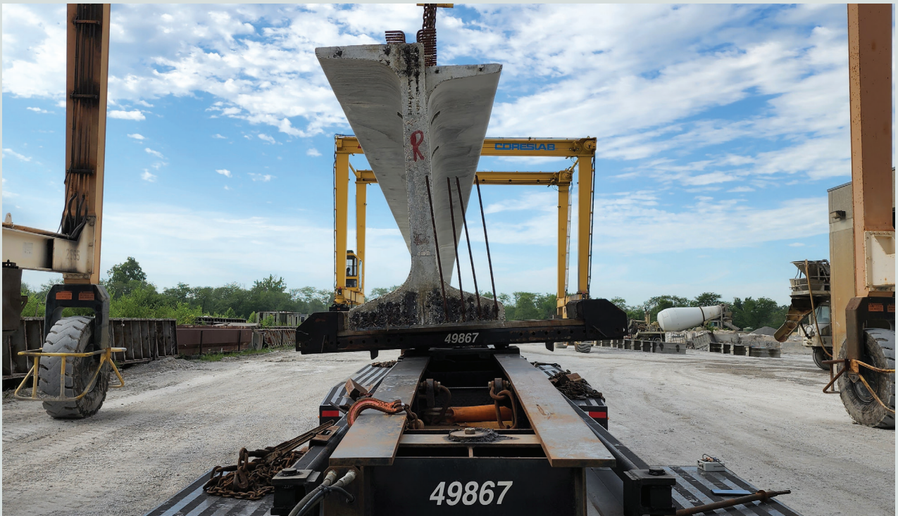
Figure 6. Girder placement on the vehicle.
