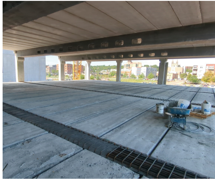
The beams and hollow-core slabs are fully erected before the topping is placed for the new Steel District office building in Sioux Falls. Courtesy of e.construct.USA, LLC.
