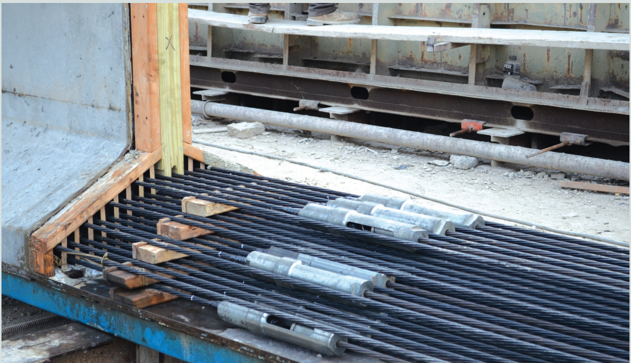
Figure 20. Coupler system to connect carbon-fiber-composite-cable strands to steel strands during prestressing.
