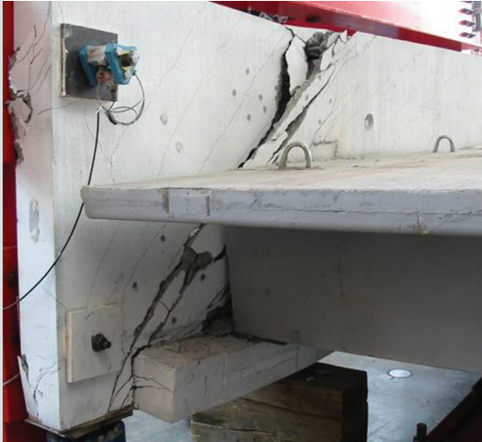
Failure mode near beam end. Source: Reproduced by permission from Lucier (2010), Fig. 3-47, p. 63.
