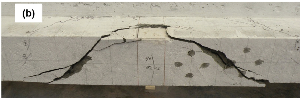
Punching shear failure mode. Source: Reproduced by permission from Rizkalla (2016), Fig. 4-15b, p. 96.
