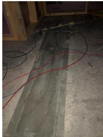
Top view of the UHPC joint between girders 2 and 3 after removing the formwork
