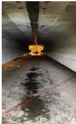
Puddles of water leaked from joint between girders 1 and 2
