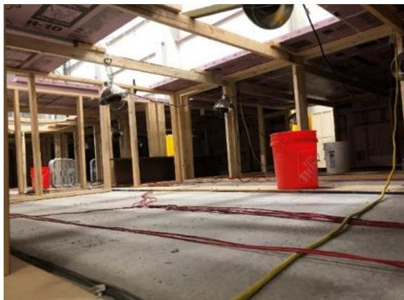
“Chimneys” at third points used to pour UHPC into the joints
