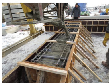
Casting of concrete mixture
