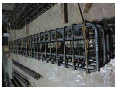
Fabrication of reinforcement cages
