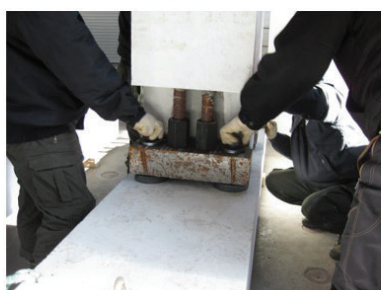
Assembly of beam and column members
