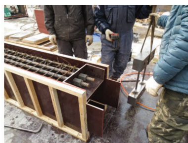
Placement of transfer block at base of beam
