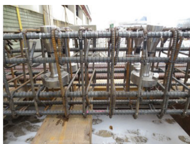
Placement of ductile rods at joint
