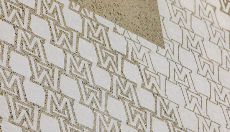
Mid-States Concrete Industries used Graphic Concrete technology to create the pattern on the low-maintenance precast concrete panels for the new Maine West High School field house. Photography by Peer Canvas.
