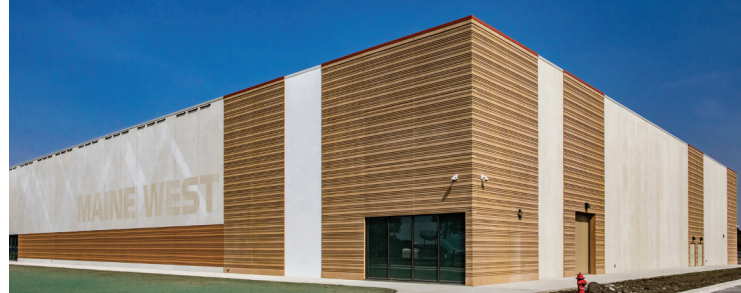
For Maine West High School’s new field house in Des Plaines, Ill., Mid-States Concrete Industries used Graphic Concrete technology to create a one-of-a-kind design. Photography by Peer Canvas.
