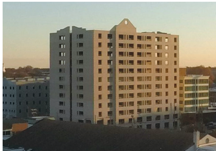
The Icon in Richmond, Va., is one of the first structures to use the new Tindall Lightweight All-Purpose Beam (T-SLAB). Courtesy of Tindall.
