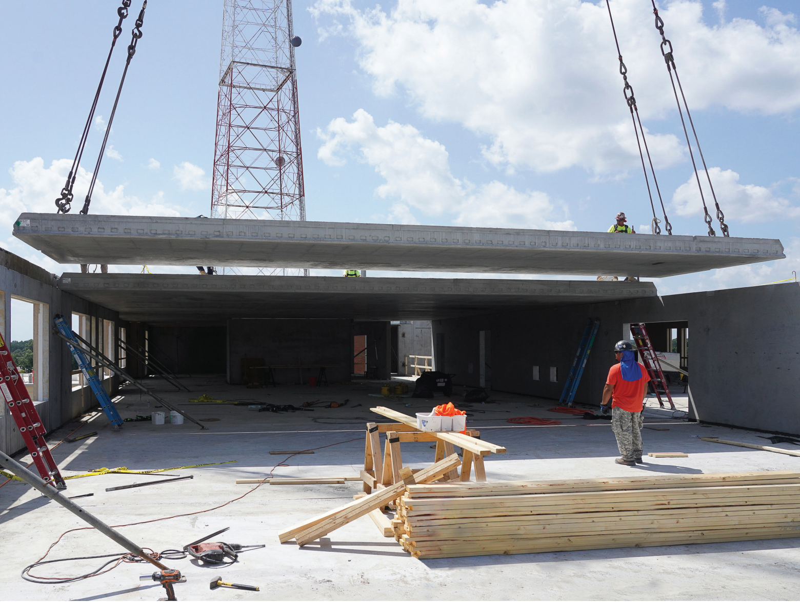
Erection of The Icon begins with Tindall Building System's T-SLAB shallow slab member. T-SLAB has spans that are relatively longer than other similar slab systems and allows for unique geometries, cast-in items, and high fire-resistance and acoustic ratings. Courtesy of Tindall.
