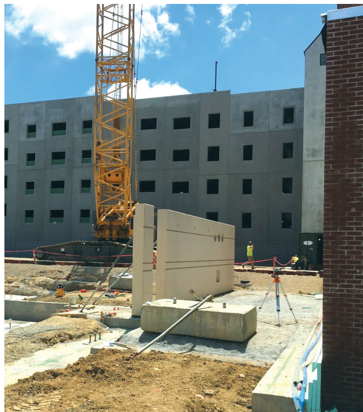
Because of the tight construction area bordered by a parking structure and adjacent to a hotel, the crane was set in the middle of the three buildings, including The Icon. Courtesy of Tindall.
