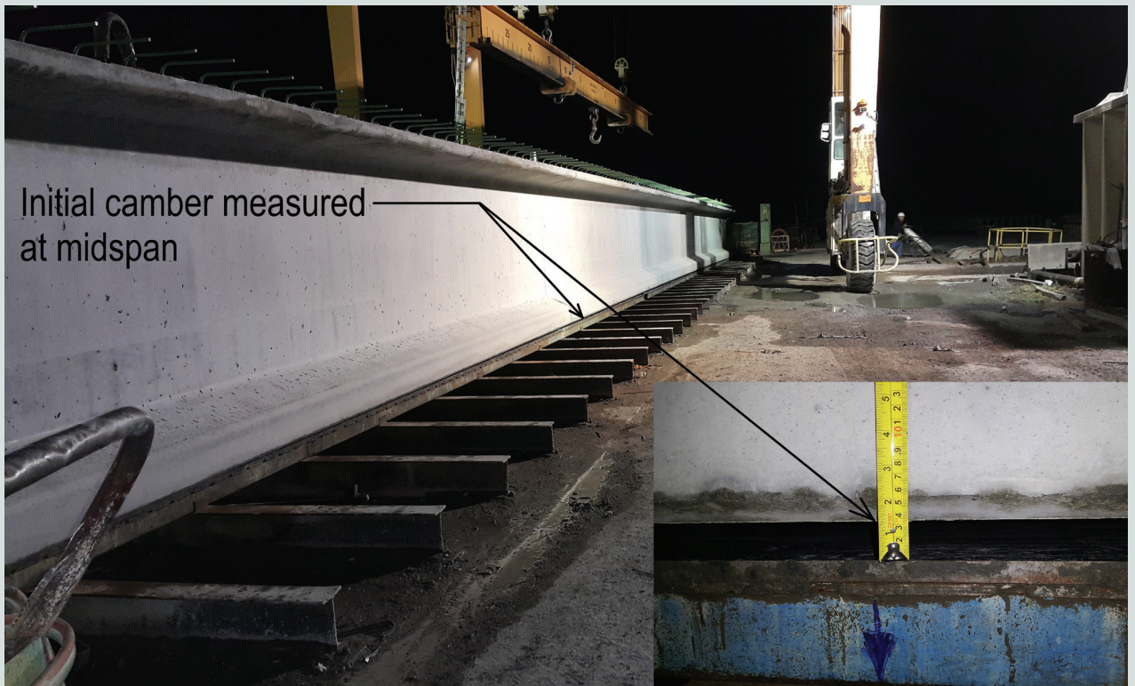
Figure 2. Initial camber measured on the casting bed.
