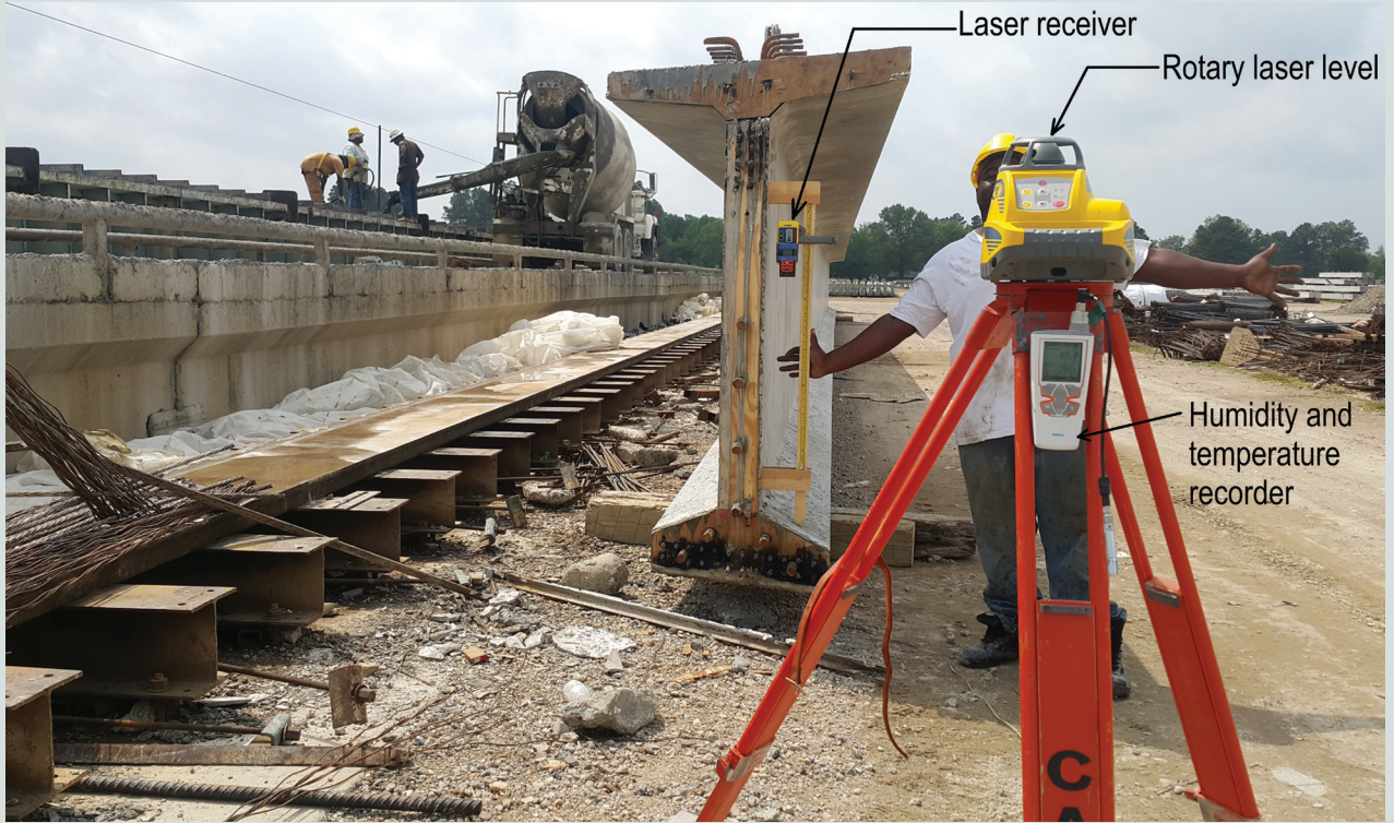
Figure 1. Rotary laser level and receiver rod used to measure camber.
