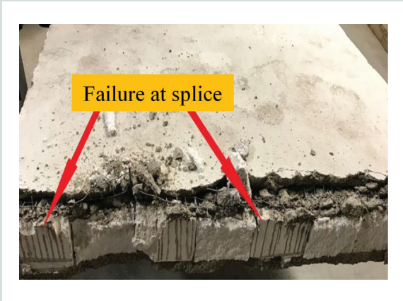
Figure 16. Typical failure plane for the medium-span specimens.
