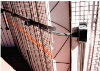
Installation of utility conduits
