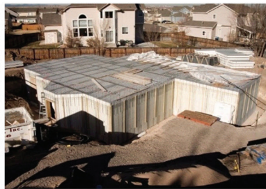
Placement of first floor
