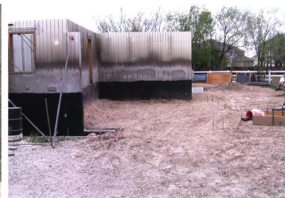
Backfilling of basement walls
