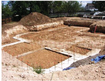
Starter reinforcing bars for the walls
