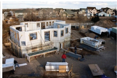
Erection of first floor walls
