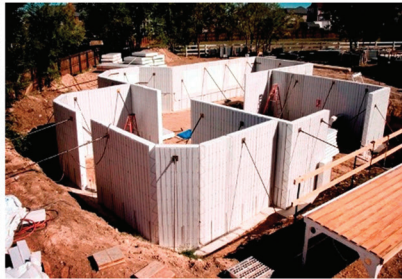
Erection of SCIP cores
