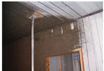
Shotcreting of interior walls and floors
