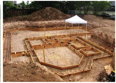
Formwork for wall footing
