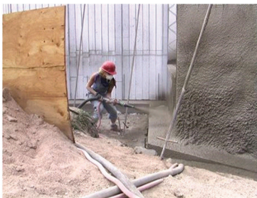
Shotcreting exterior walls
