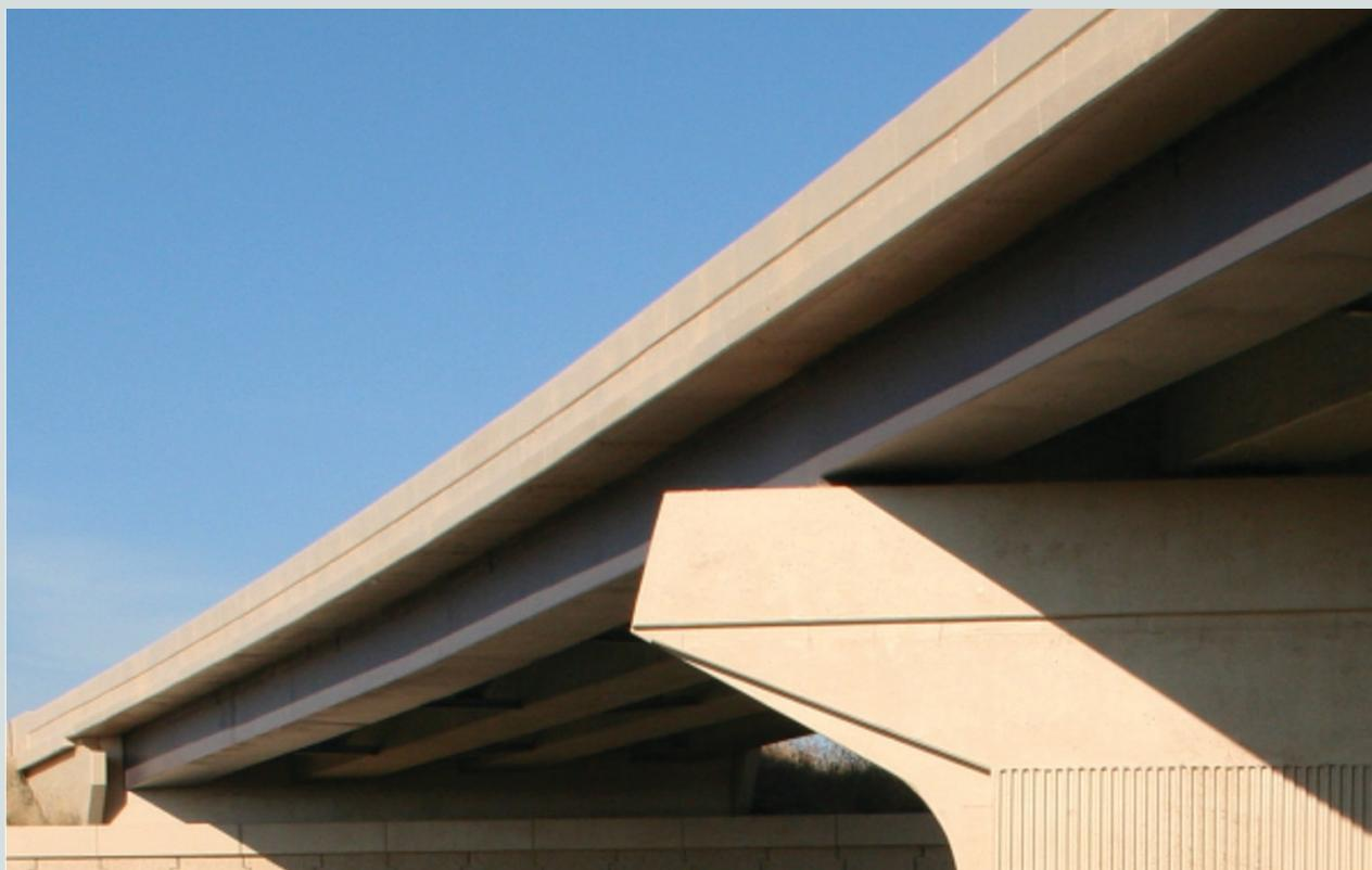
**Figure 1.** Arbor Road over Interstate 80 bridge near Lincoln, Neb. The curved alignment was made with straight, chorded 40 ft long segments. Source: Reproduced from Sun et al. (2007). Note: 1 ft = 0.305 m.
