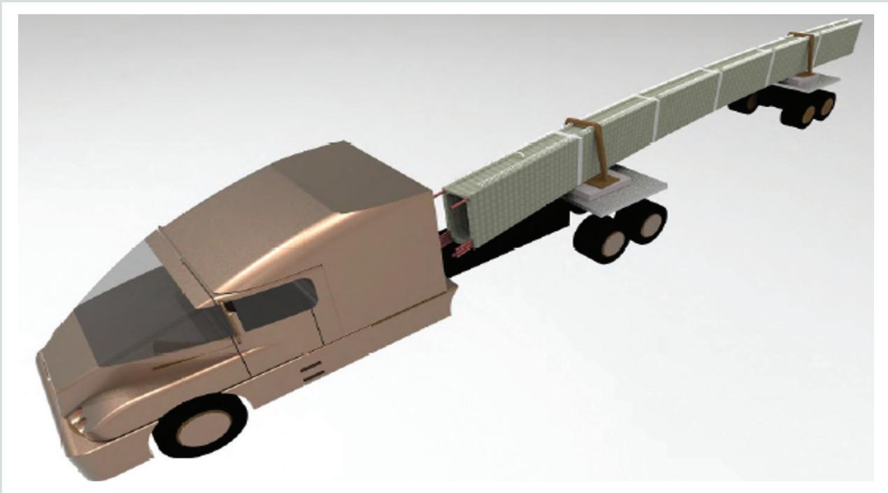
**Figure 8.** Transporting the six-girder assembly.
