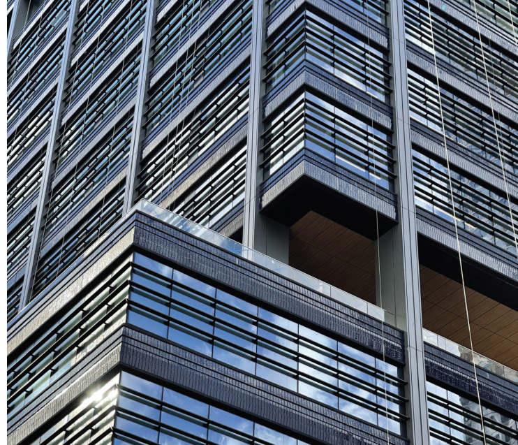
Cobalt blue glazed brick on precast concrete spandrels gives One Willoughby Square in downtown Brooklyn, N.Y., a distinctive, high-end look. Courtesy of Michael Young.
