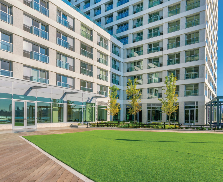
The Beach residential apartments' thick precast concrete exterior, provided by Architectural Precast Innovations Inc., helped meet the building's energy model requirements with the hollow-core by Nitterhouse contributing to floor and roof building codes. Courtesy of Newport Leasing Office.
