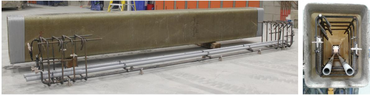
Polyvinyl chloride ducts and steel cages
