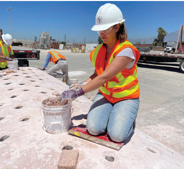
University of Southern California architecture student Rachel Hamilton applies a skim coat to the precast concrete around the openings in the panels of the Carapace Pavilion. All photos courtesy of Douglas Noble.
