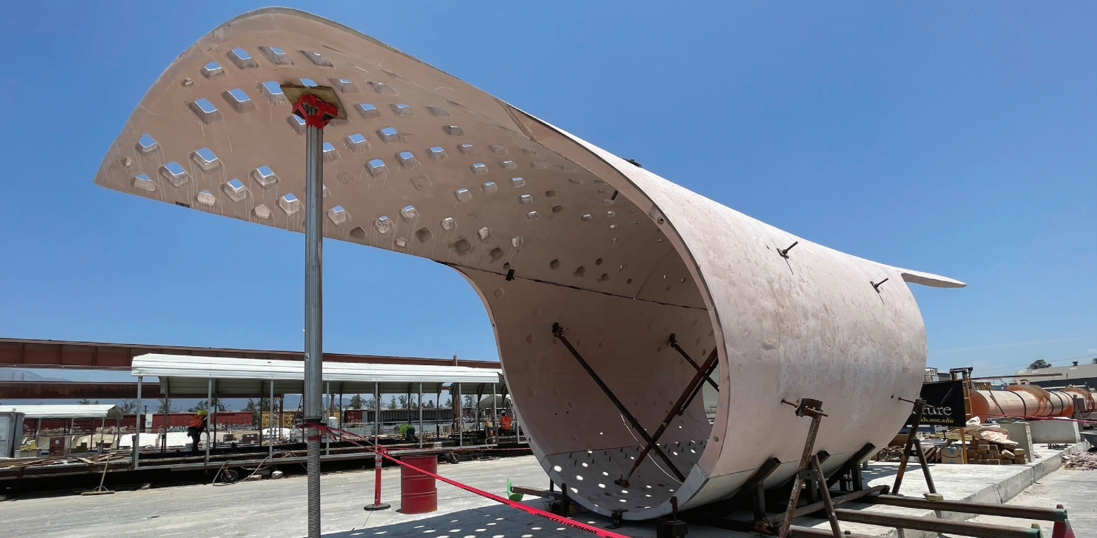
The Carapace Pavilion waits, prior to cleaning, in the Clark Pacific casting yard in Fontana, Calif., to be installed at Joshua Tree National Park. The structure is 42 ft (13 m) long overall and 13 ft (4 m) tall. The steel fiber reinforcement in the ultra-high-performance concrete will rust and streak over time, helping the structure's colors blend into the natural environment.
