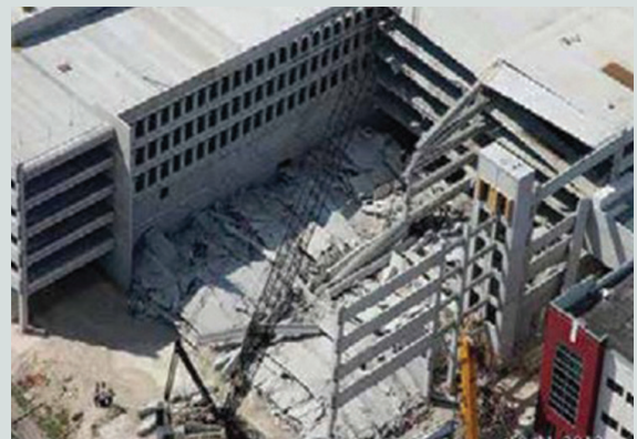
Figure 7. View of the Miami, Fla., parking structure collapse. Courtesy of Occupational Safety and Health Administration.
