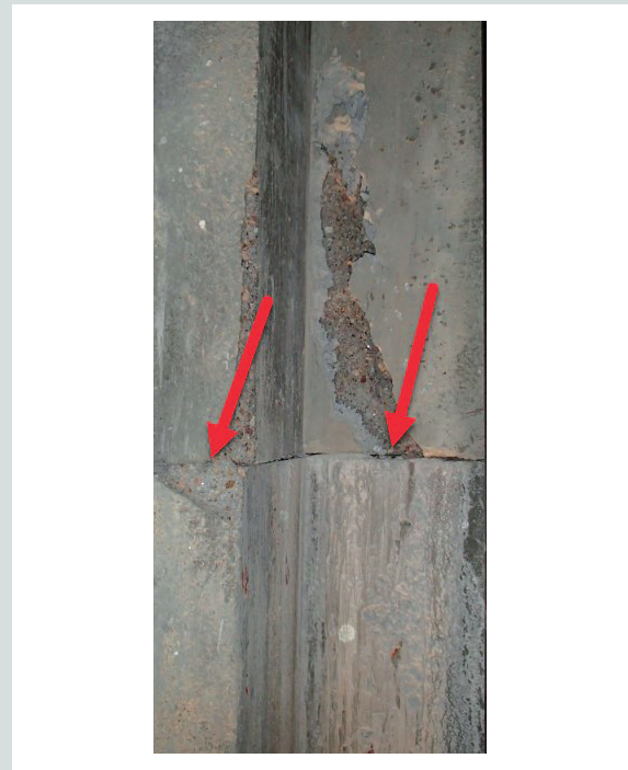
Figure 5. Horizontal wall-to-wall joint sudden closure—no grout.
