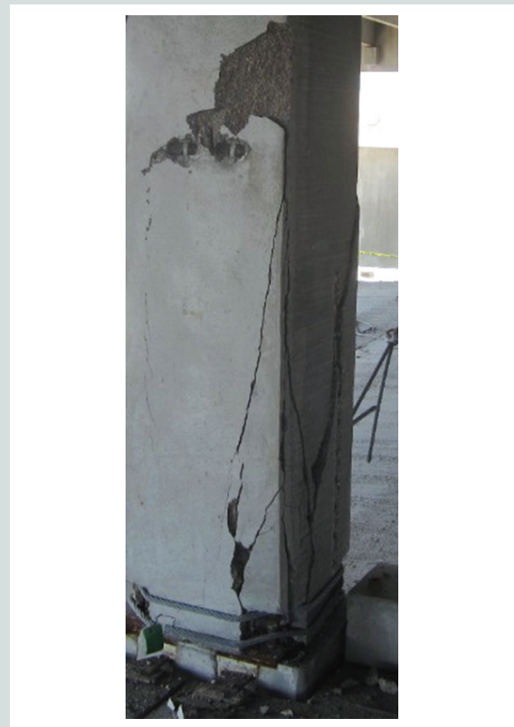
Figure 6. Failure of precast concrete column—no grout.
