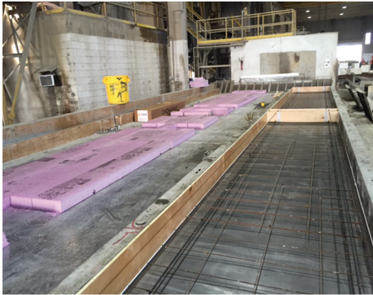
Forms with outer wythe reinforcement installed
