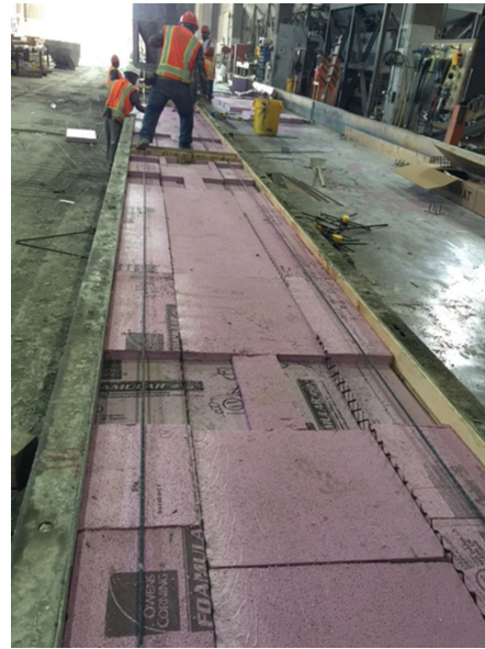
Foam core with carbon-fiber-reinforced polymer grid installed after casting the outer wythe
