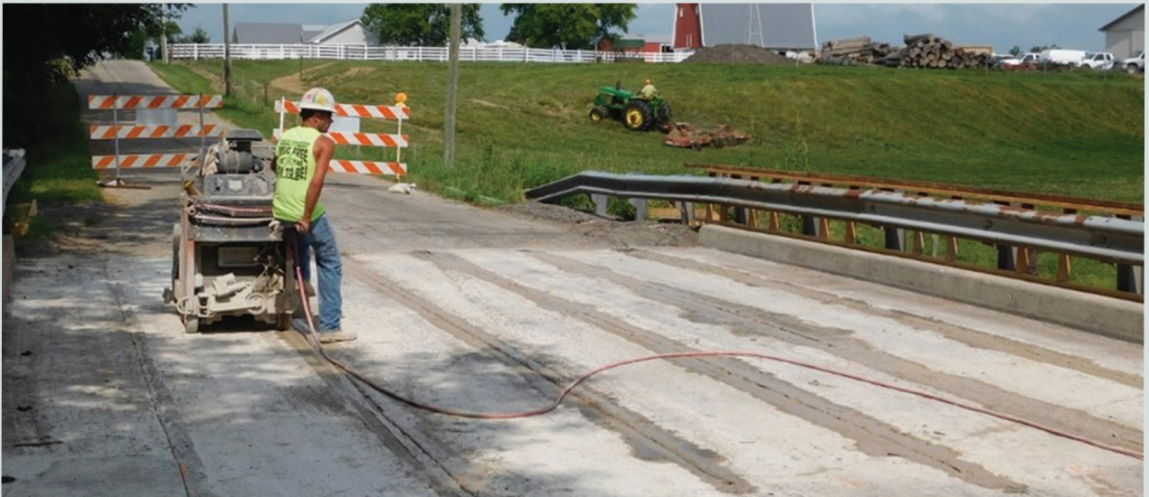
Figure 7. Shear key-cutting operation.
