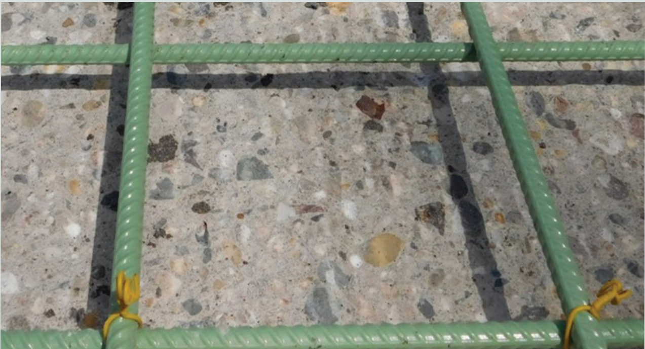
Figure 8. Sandblasted box-beam surface.
