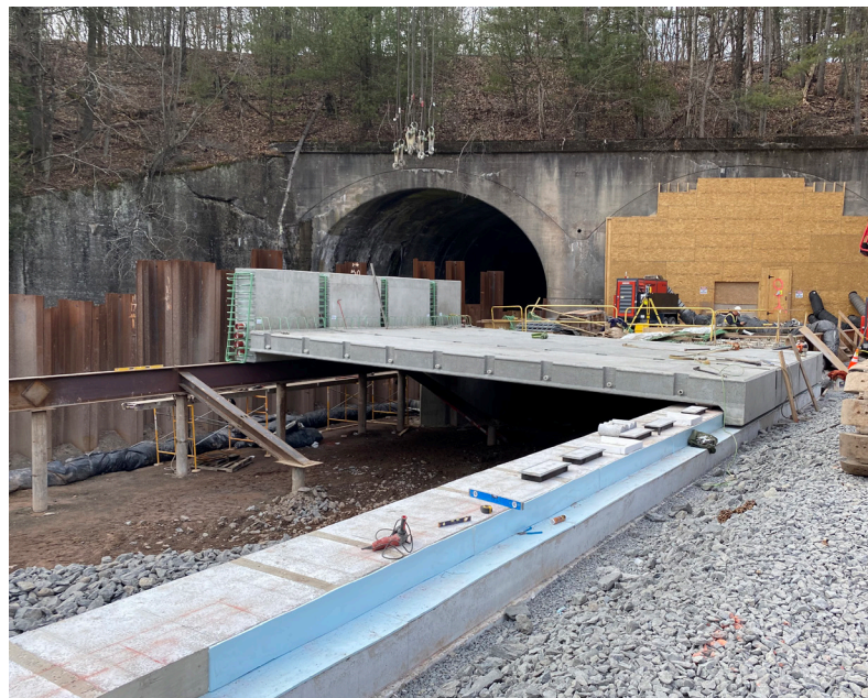
The new State Route 191 bridge replacement project inside Stites Tunnel includes a 345 ft (105 m) long precast concrete box culvert structure inside the tunnel and two new post-tensioned precast concrete approach spans. Photo by Larson Design Group.
