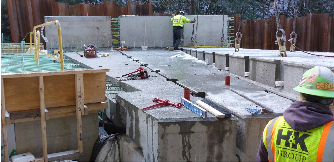
The north approach span of the new State Route 191 bridge replacement inside Stites Tunnel in East Stroudsburg, Pa., includes two tapered precast concrete segments. Photo by Larson Design Group.
