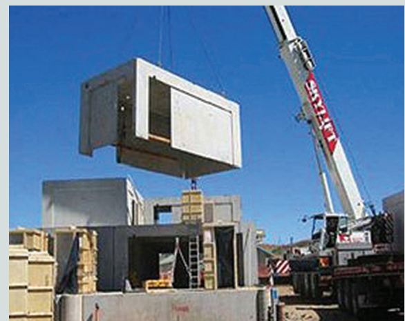
Figure 6. Precast concrete module being placed. Courtesy of Doug Buhrens.
