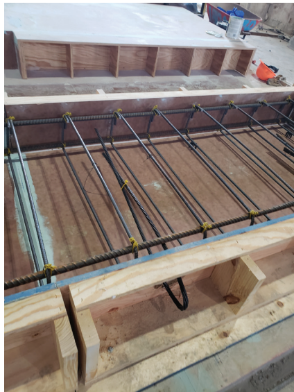
Straight lifting loop in place prior to casting
