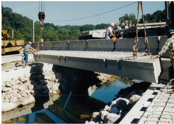
Bridge beam suspended from crane with lifting loops
