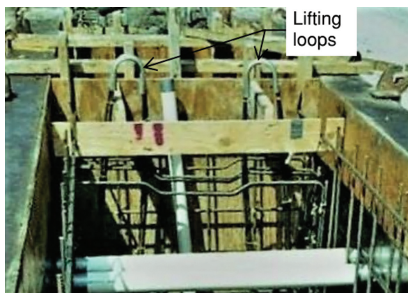
Lifting loops prior to concrete casting
