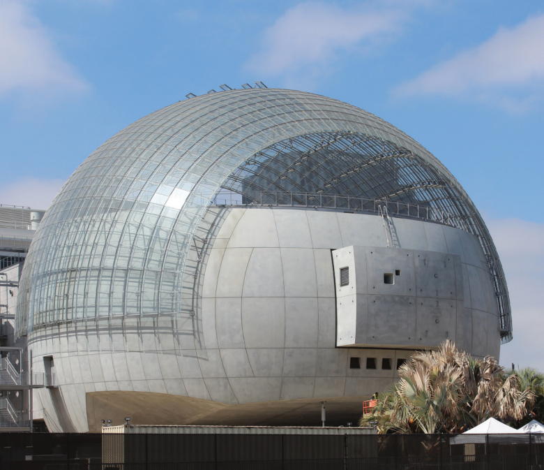
The new Academy Museum of Motion Pictures in Los Angeles, Calif., includes a 60,000 ft 2 (5600 m 2 ) spherical glass and concrete structure to house a 1000-seat theater. It originally was planned as a cast-in-place concrete shell but was converted to precast concrete. Courtesy of Willis Construction Inc.
