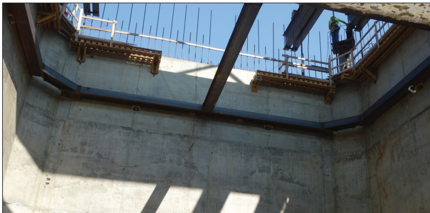
Figure 21. View from underneath the lifted cofferdam. Reproduced by permission from the U.S. Army Corps of Engineers.
