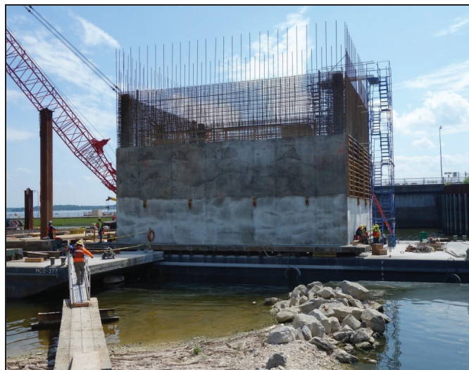
Figure 2. Casting of the precast concrete cofferdam on the casting barge. Photo courtesy of Johnson Brothers Southland Holdings.
