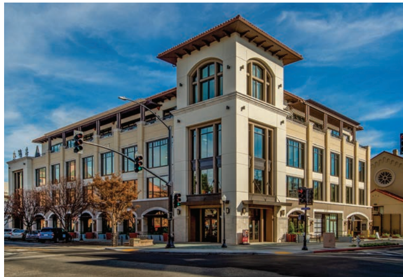
The mixed-use 599 Castro project in Mountain View, Calif., uses glass-fiber-reinforced precast concrete to help maintain the Mission style architecture in the area. Courtesy of ARC TEC Inc.
