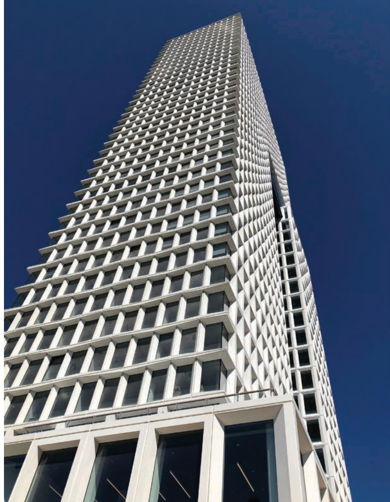
Gate Precast Co. received the 2020 Sidney Freedman Craftsmanship Award for One South First in Brooklyn, N.Y. Courtesy of Gate Precast Co
