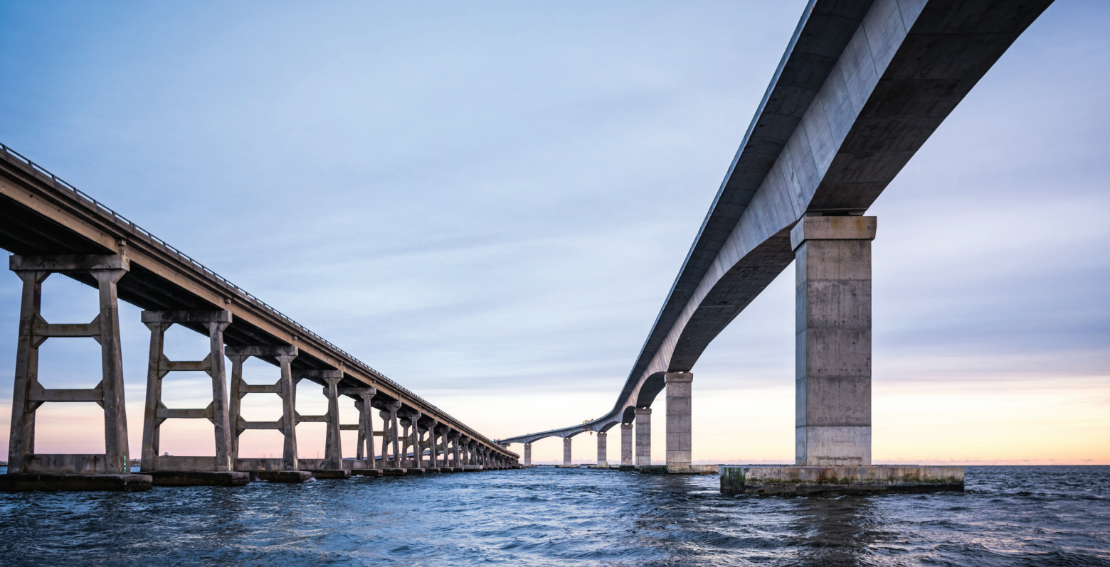
The Marc Basnight Bridge, right, along the North Carolina coast won a 2020 PCI Sustainable Design Award. It replaces the Bonner Bridge, left, which opened in 1963, and most of which will be demolished. Photo courtesy of HDR Inc.: © 2019.
