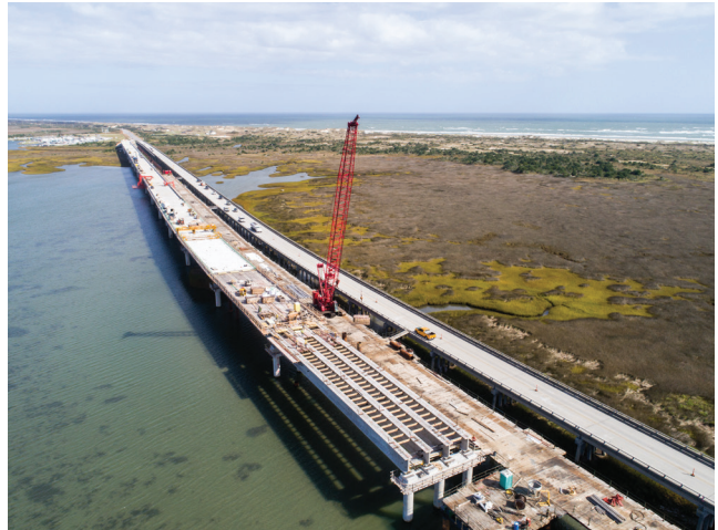
To withstand the saltwater environment, stand up to hurricane winds, protect vulnerable species, and achieve a 100-year service life, the Marc Basnight Bridge in North Carolina was constructed with precast concrete. Photo courtesy of HDR Inc.: © 2019.
