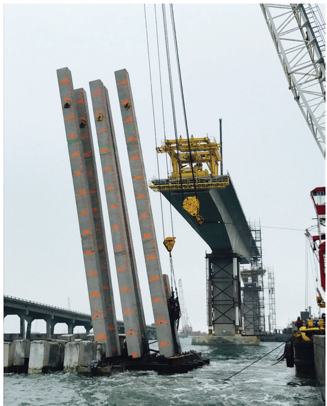
Construction of the Marc Basnight Bridge in North Carolina was a dangerous feat with treacherous currents, constantly shifting depths, and high winds. Photo courtesy of HDR Inc.: © 2019.
