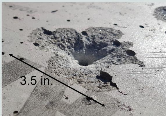
**Figure 4.** Back-face concrete blowout due to drilling.
