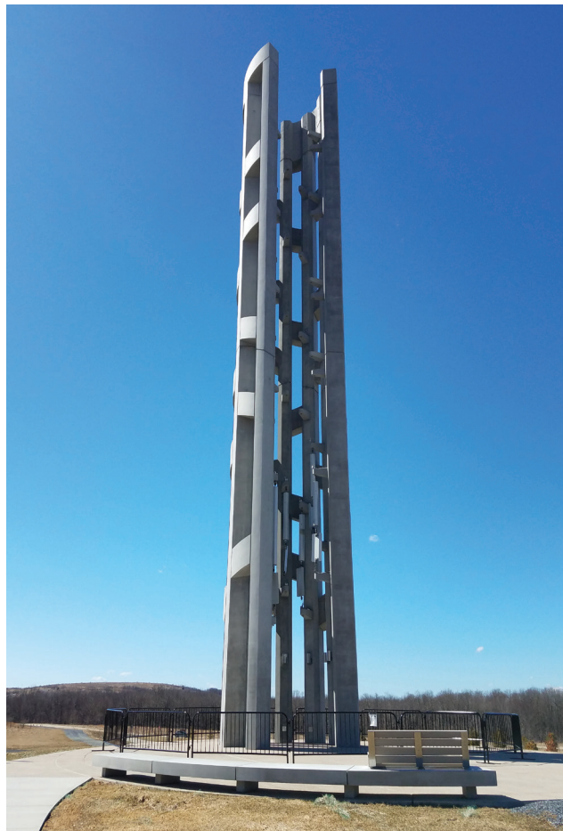
Integrating BIM and precast concrete enabled the precision necessary to use only internal connections in this precast concrete memorial to the passengers and crew of United Flight 93, which crashed in Somerset County, Pa., on September 11, 2001. Courtesy of Brenda Torrey, Friends of Flight 93.
