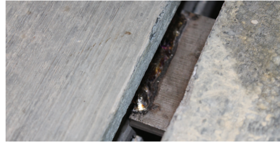
Erection bar after welding
