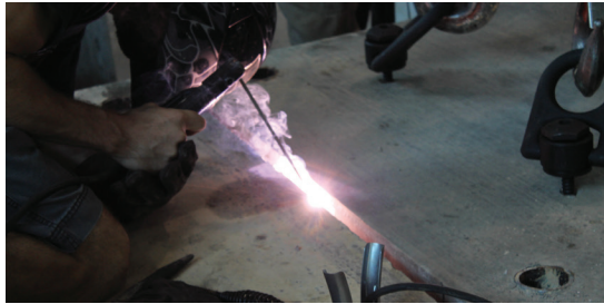
Welding the erection bar to the test panel
