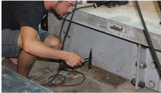
Welding the erection bar to the fixed panel
