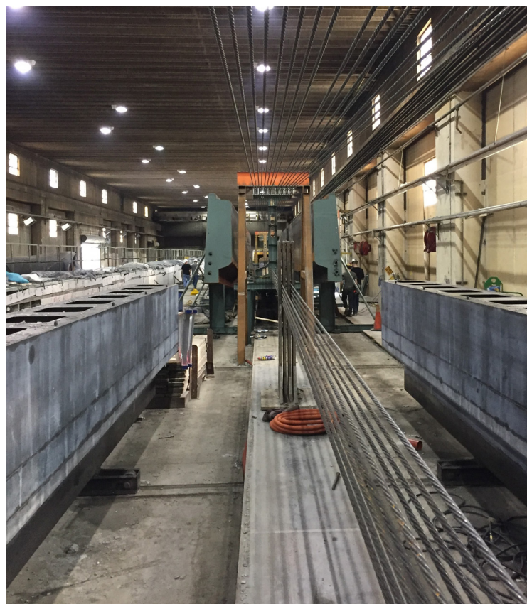
Some beams for the Lehigh Valley Bridge are as deep as 10 ft, requiring the prestressing strands for the top flange to be positioned much higher than usual. Photo by Gary Lehman.
