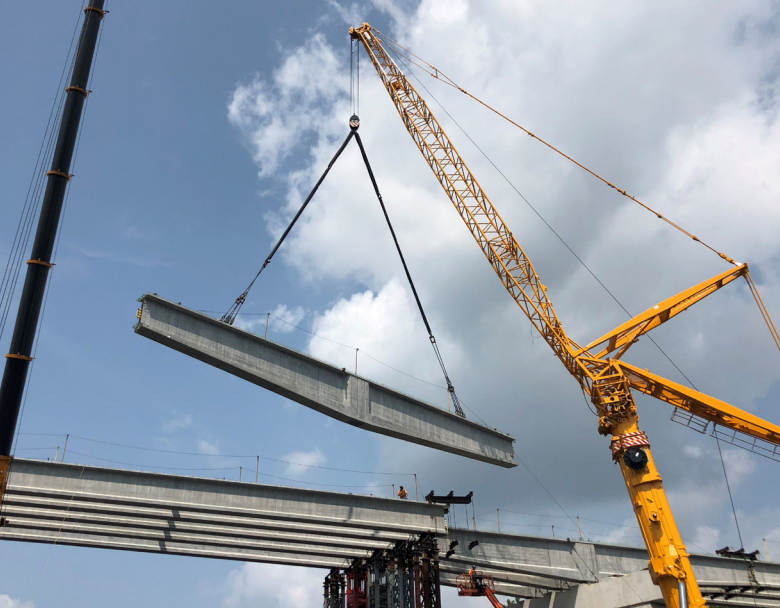
A prestressed and post-tensioned bulb-tee beam is being lowered into place for the Lehigh Valley Bridge. Northeast Prestressed Products LLC of Cressona, Pa., manufactured and installed the precast concrete elements used in the project. Photo by Danielle M. Fleagle.
