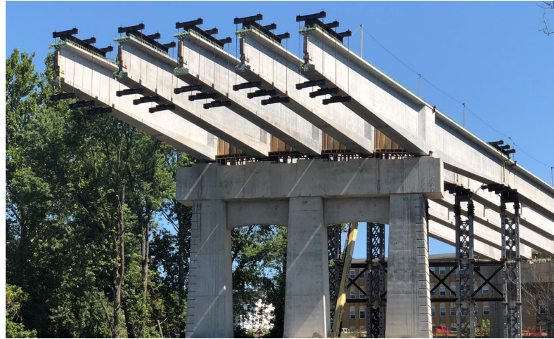
The Lehigh Valley Bridge uses spliced girders to support bulb-tee beams. Photo by Danielle M. Fleagle.
