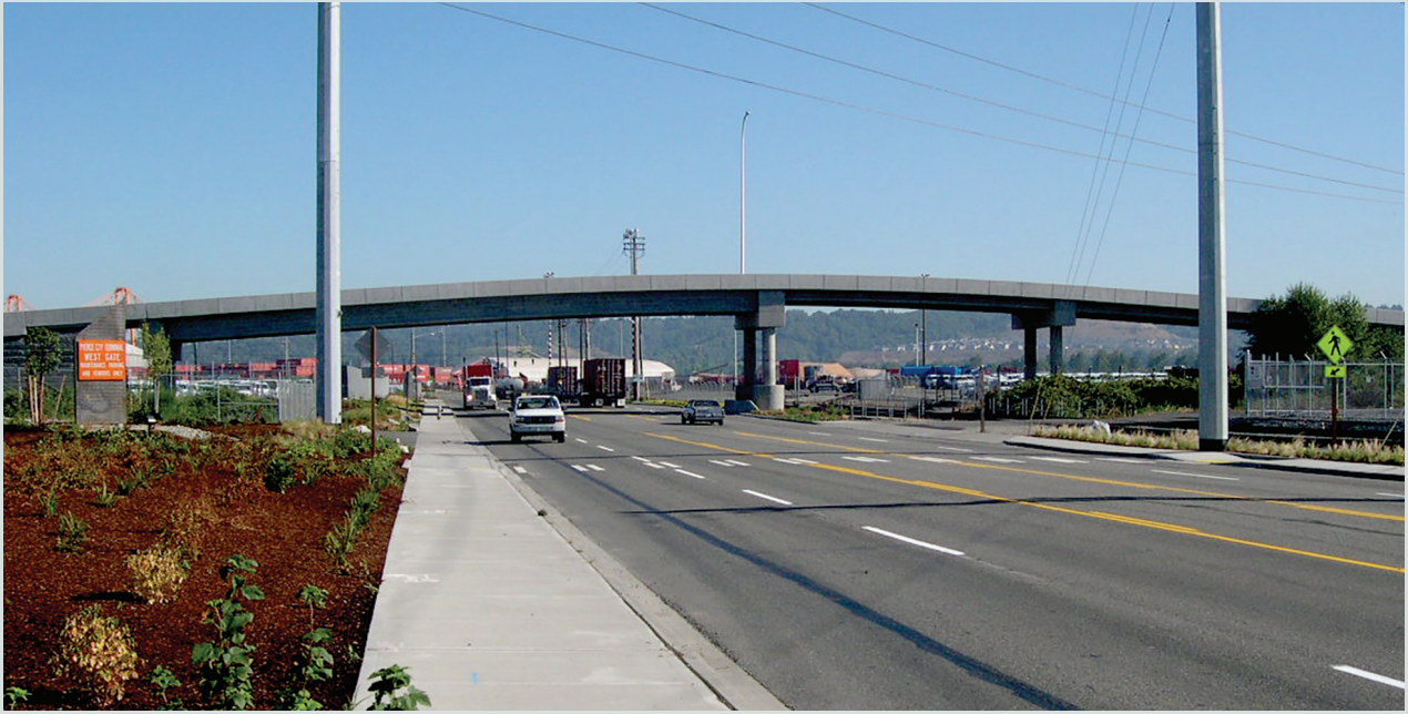
Figure 13. Marshall Avenue Bridge with variable precamber in the main span. Courtesy of Concrete Technology Corp.
