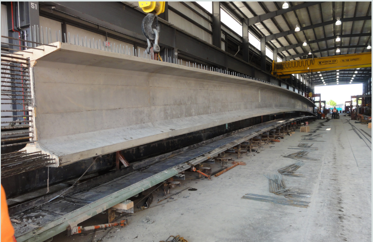
Figure 4. Stripping a precambered girder from the form.
