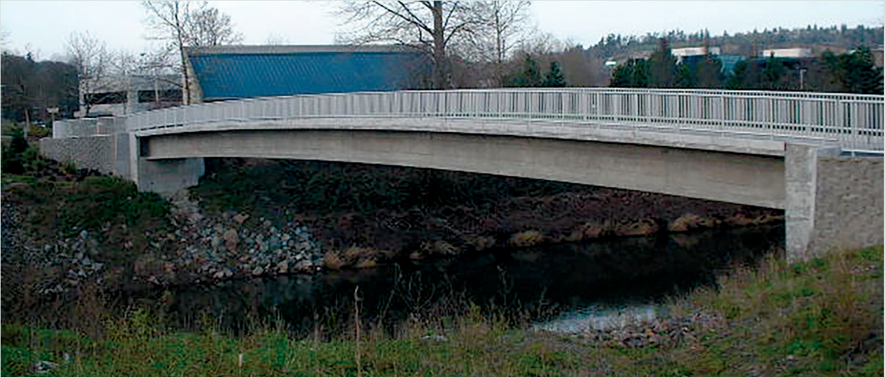
Figure 11. Completed Interurban Trail Pedestrian Bridge. Courtesy of Concrete Technology Corp.
