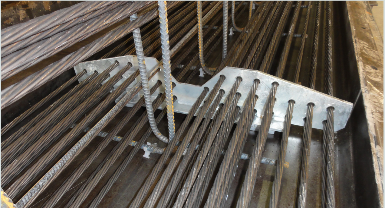
Figure 3. Straight strand deviator plate in precambered girder.
