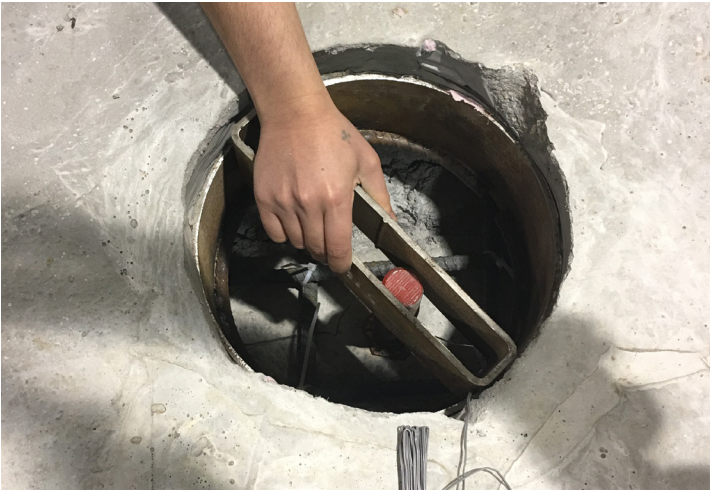
Placing the inner HSS around the shear connector
