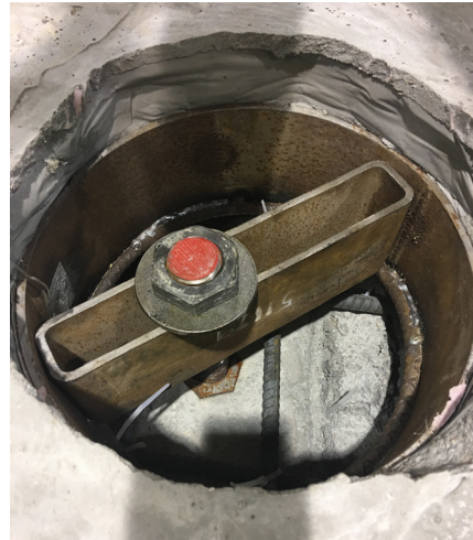
Installing the washer and nut (snug tight)
