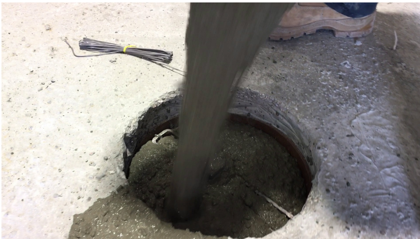
Placing SCC in the shear pocket and haunch
