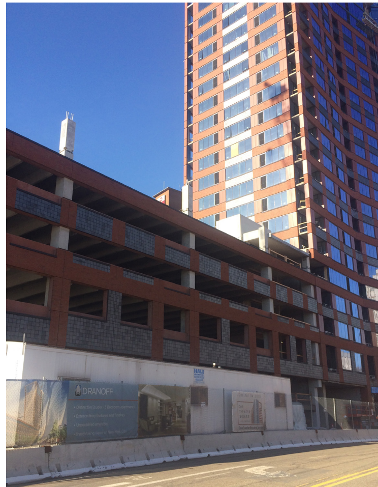
The parking portion of the $94 million One Theatre Square in Newark used 237 pieces of precast concrete. Courtesy Architectural Precast Innovations.
