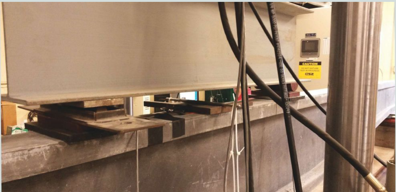
Figure 3. Experimental test setup with steel spreader beam, rollers, and pads for beam configuration 3.
