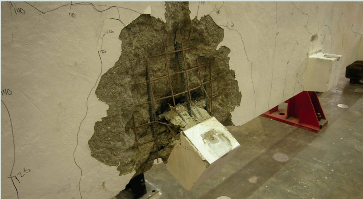
Figure 6. Corbel failure of specimen SP19.
