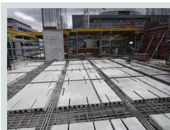
Figure 1. Construction of an untopped hollow-core diaphragm incorporating connection details in broken cores. Photo courtesy of Manufacturas de Cemento SA.
