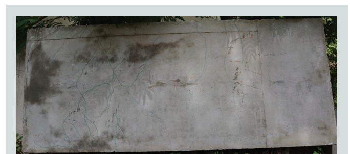
Figure 6. Cracks in bottom wythe of panel PB. Note: PB = panel tested in bending.
