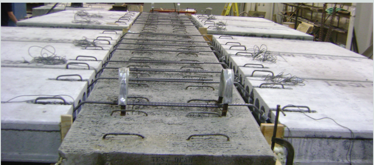
Figure 9. Installation of beam-hollow-core connection reinforcement.
