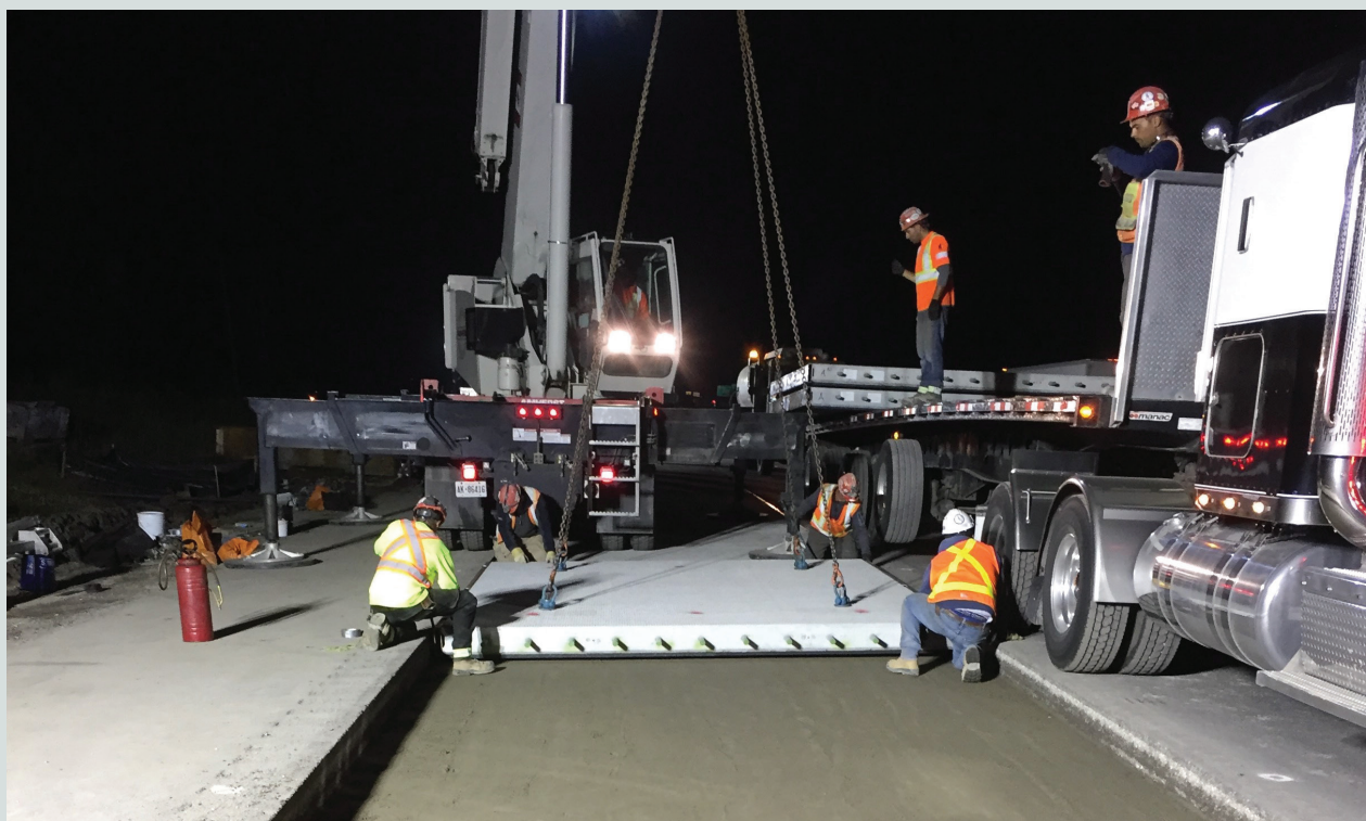
Figure 1. Installation of a precast concrete inlay panel during trial section construction.
