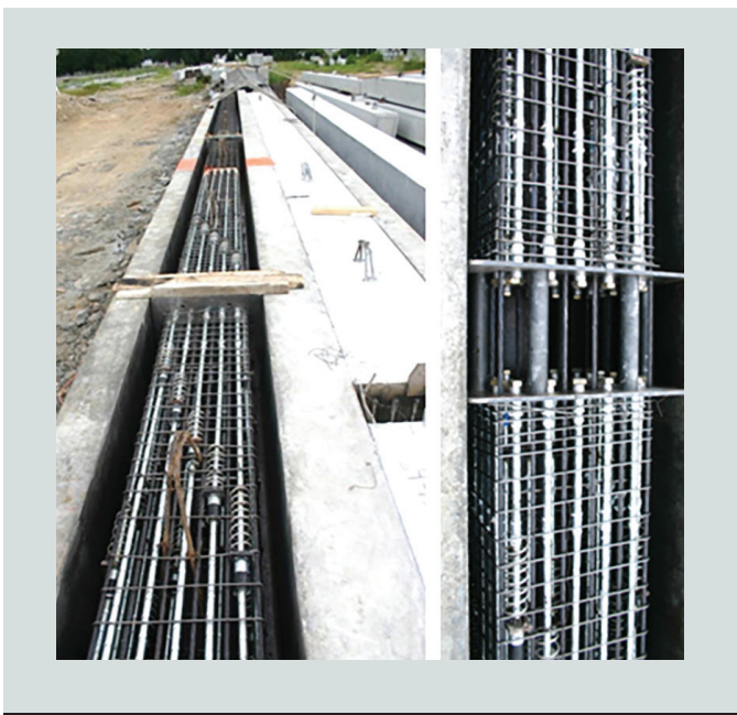
Figure 4. Fully stressed bed with lifting hooks (left) and splicing header connection (right).
